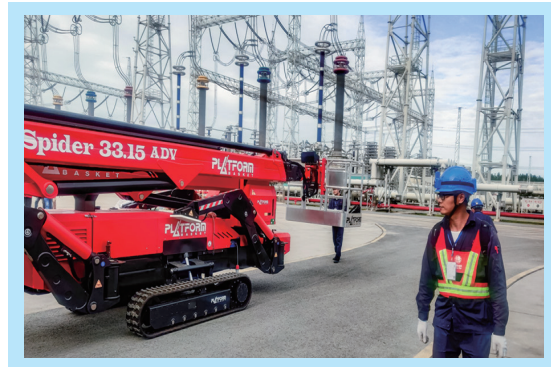
Power Equipment Inspection FIG6
